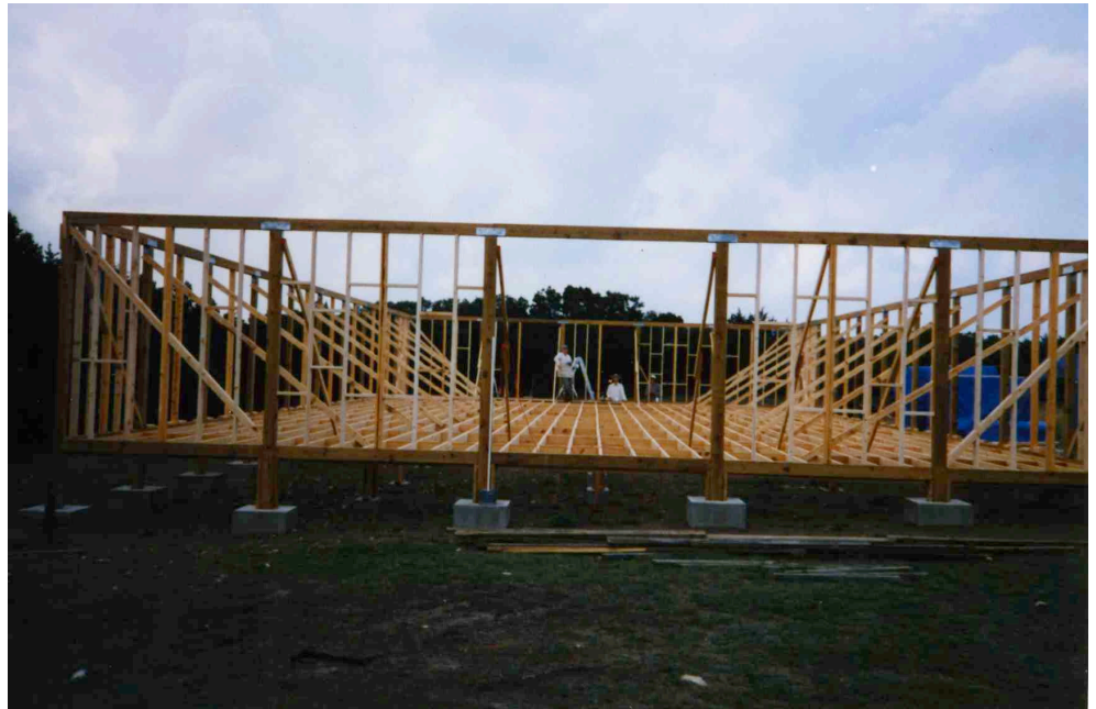
Frame goes up, gets filled in and braced up.
